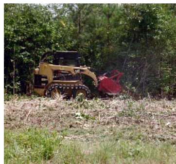
Skid-steer mulcher preparing site.
