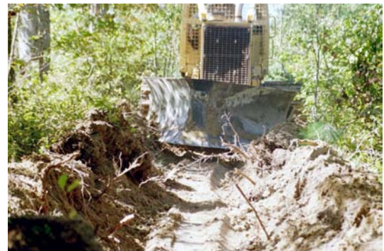
Virginia Department of Forestry installing firebreaks.
