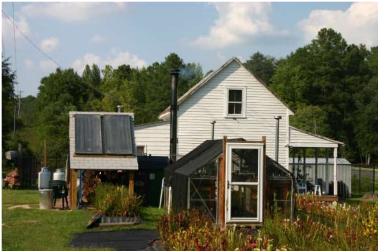
Figure 7. Outside wood furnace and hot water solar panels provide domestic hot water and heat facilities at Meadowview.
