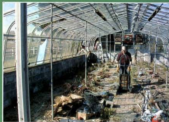
Ed Trombley removes masonry from greenhouse
